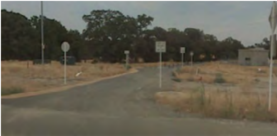
Entrance to shared driveway/ trail on Woodcreek Oaks Blvd.
