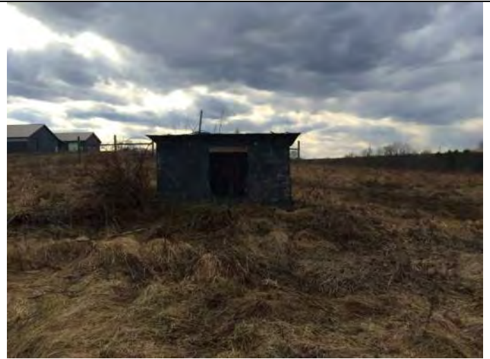
Electrical structure on eastern central portion of Site
