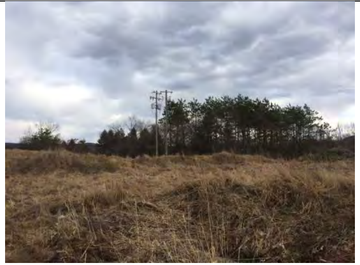
Pole-mounted transformer on eastern portion of Site
