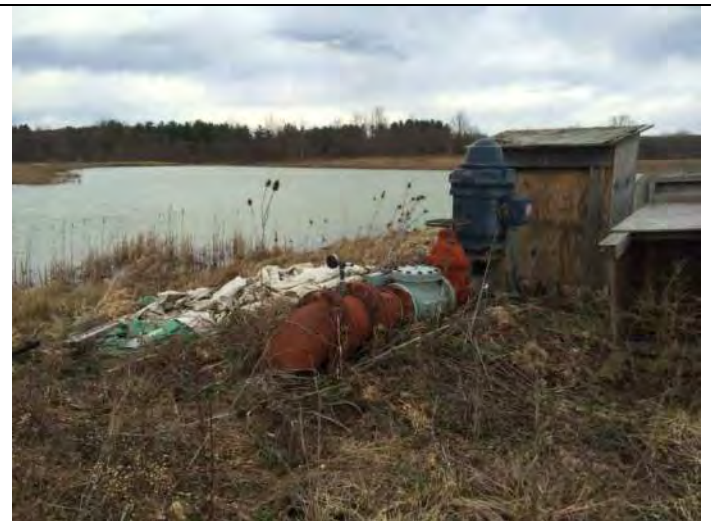
Water pump associated with northern adjacent retention pond
