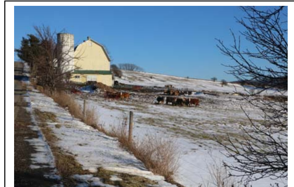
Farm along McClintock Road in winter. The barn has a steel frame and was built in 1908 by the Groton Bridge Co. It is unique. Peter Davies
