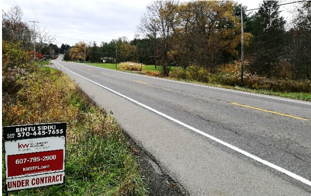
View east along Slaterville Road.
