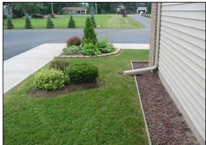
Figure 5.37 Disconnection of rooftop to designated vegetated areas. Otter Creek, NY, NYSDEC.
