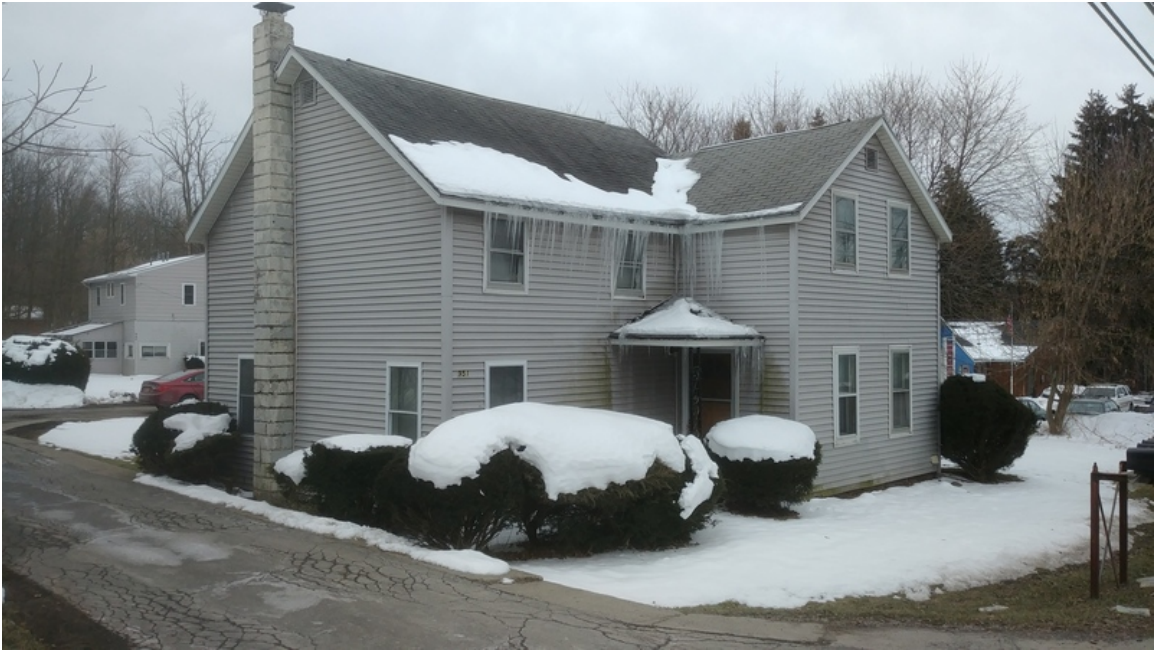
Photo 13: 951 Dryden Road facing southwest (2 units)
