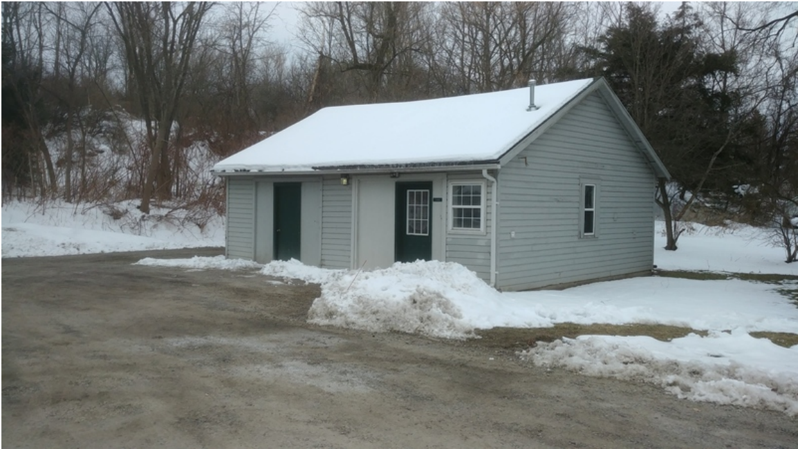
Photo 2: Laundry room and maintenance shop on 959 Dryden Road
