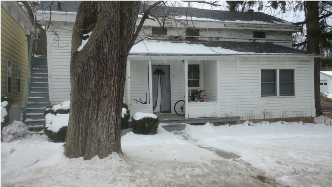
Photo 10: 957 Dryden Road units A and B
