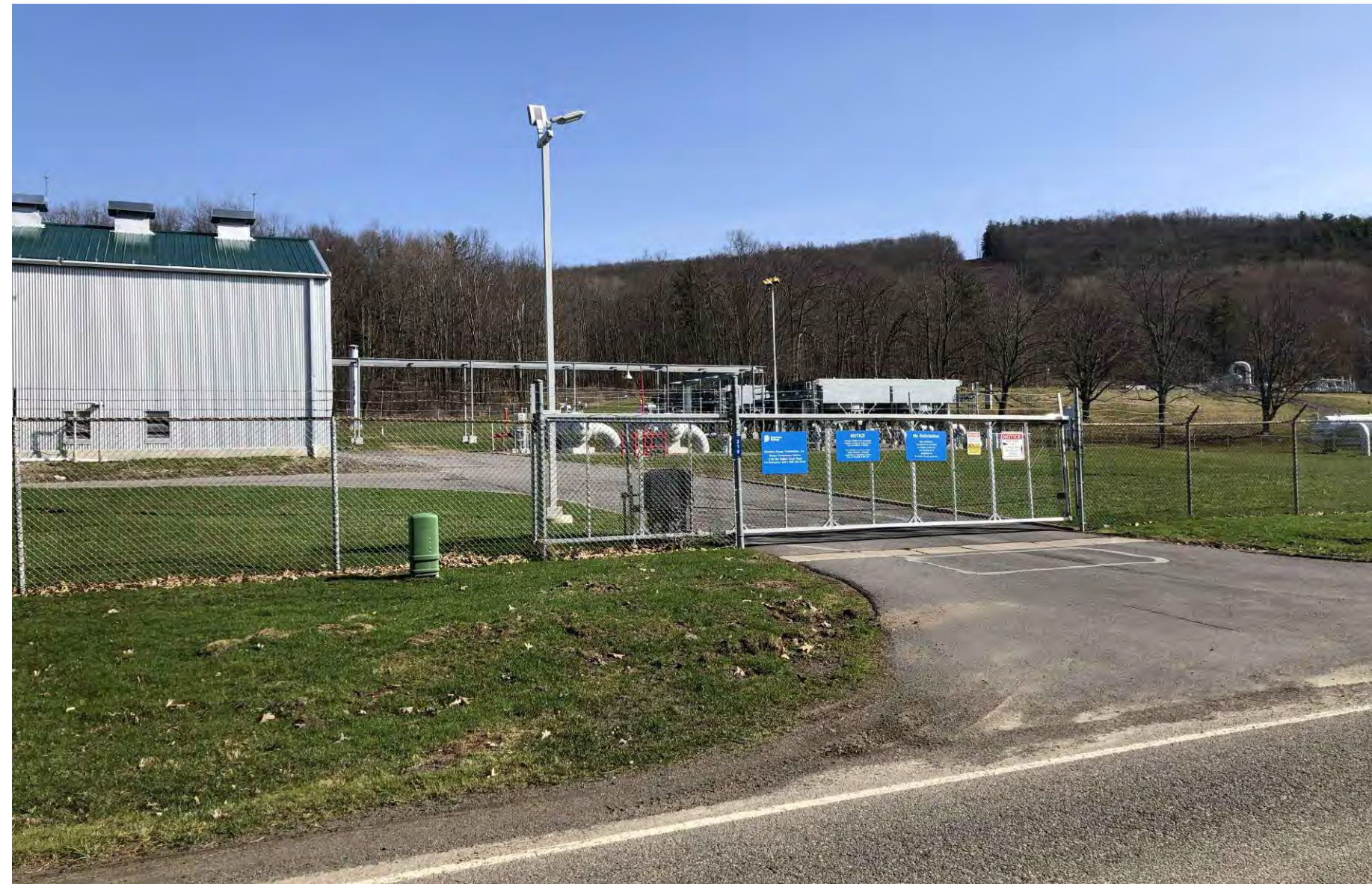
VIEW NO 6 - EXISTING CONDITIONS
