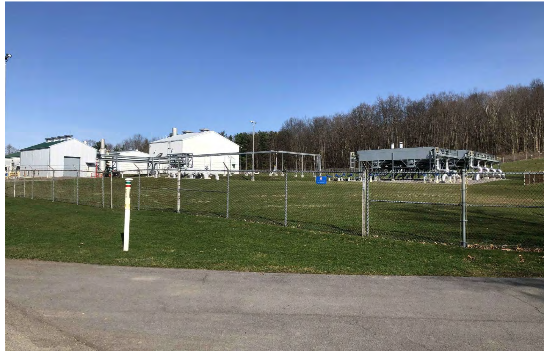
VIEW NO 2 - EXISTING CONDITIONS
