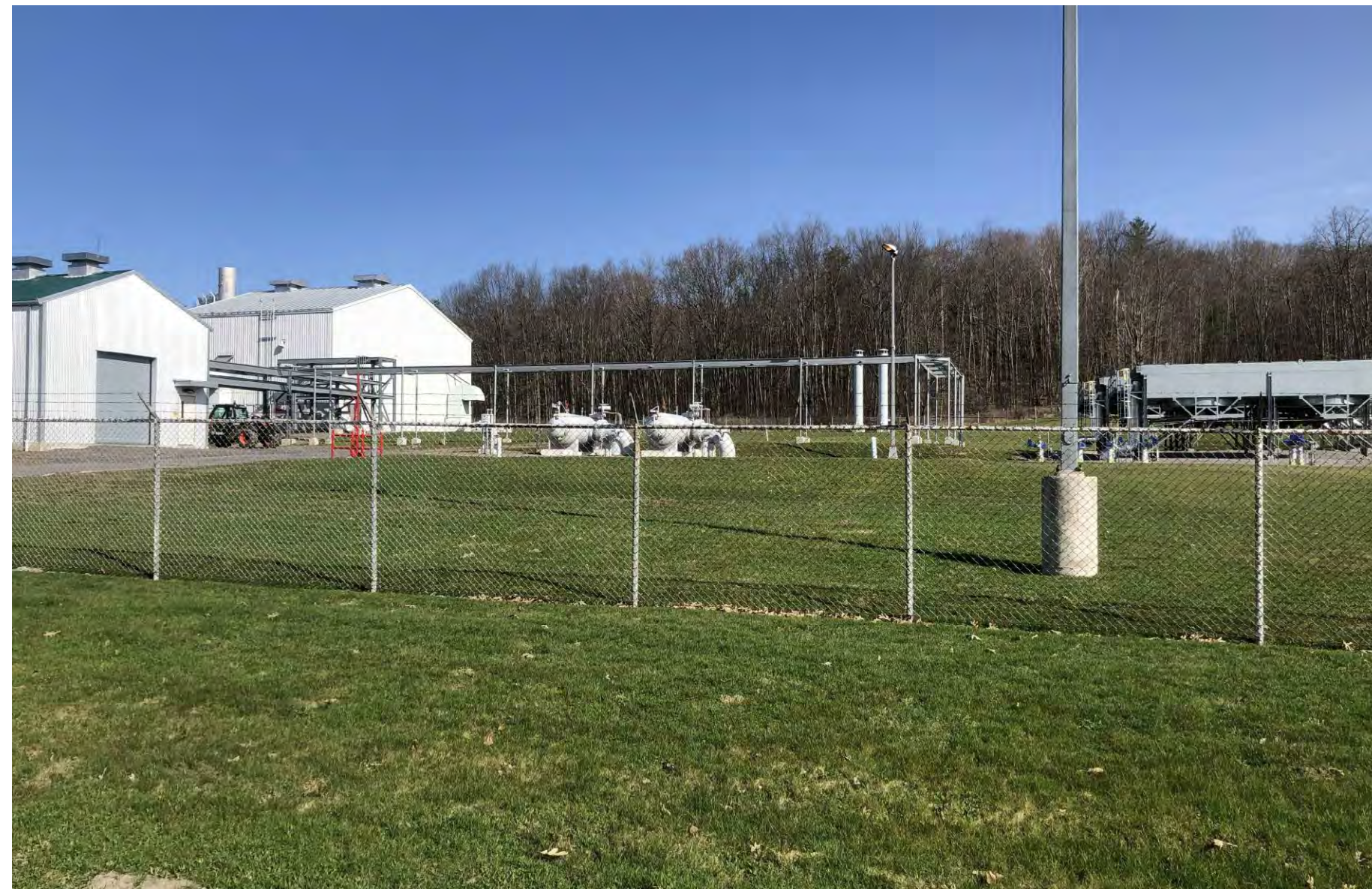
VIEW NO 3 - EXISTING CONDITIONS
