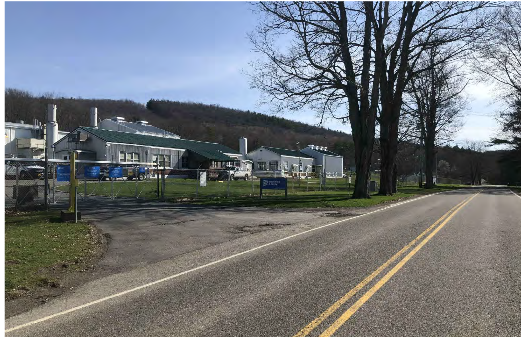
VIEW NO 4 - EXISTING CONDITIONS
