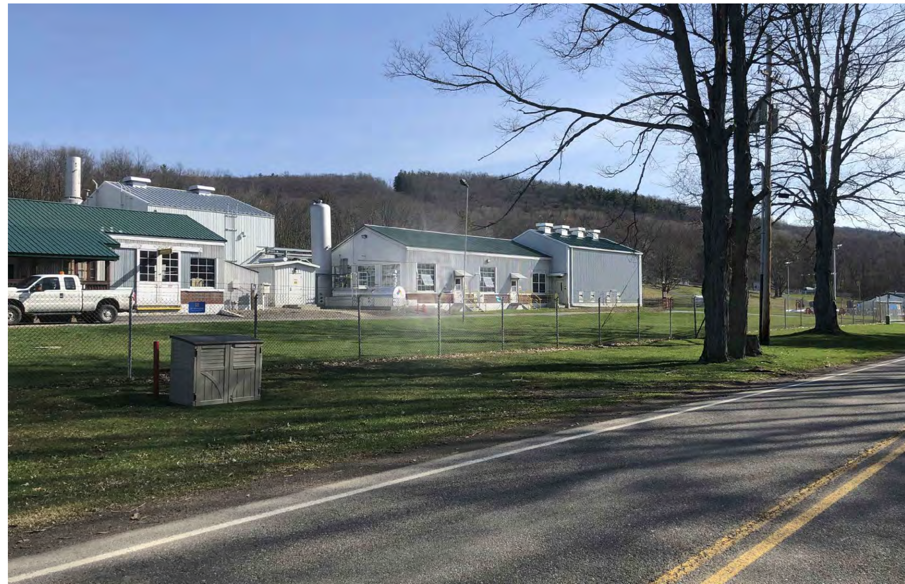
VIEW NO 5 - EXISTING CONDITIONS
