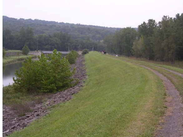
Figure 5.4.4-1. Cayuga Inlet Levee System
