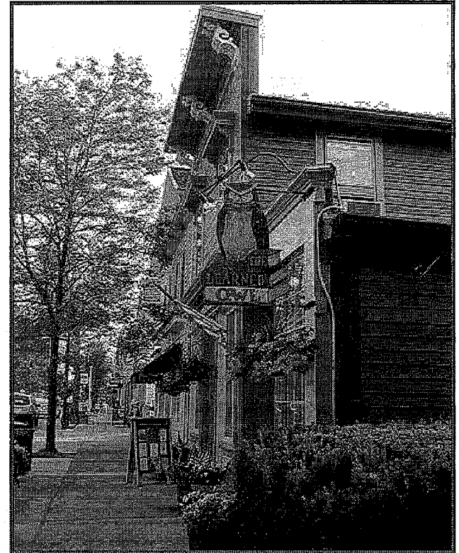
Buildings should maintain a "human scale" where height and size are proportional to human height.
