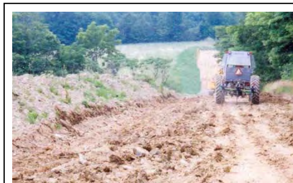
Fig. 1. A typical deep ripping phase of this practice, during the first in a series of progressively deeper “rips” through severely compressed subsoil.
