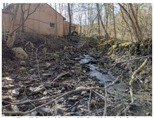
Photo 12: Streambank Erosion at 9 Knollwood Drive – Facing South
