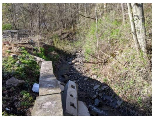
Photo 5: Failing Concrete Wall at 6 Knollwood Drive
