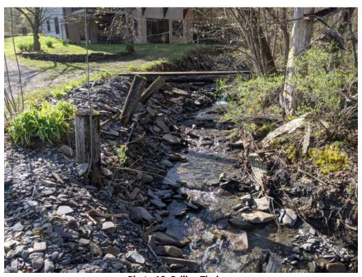
**Photo 10: Failing Timbers**
