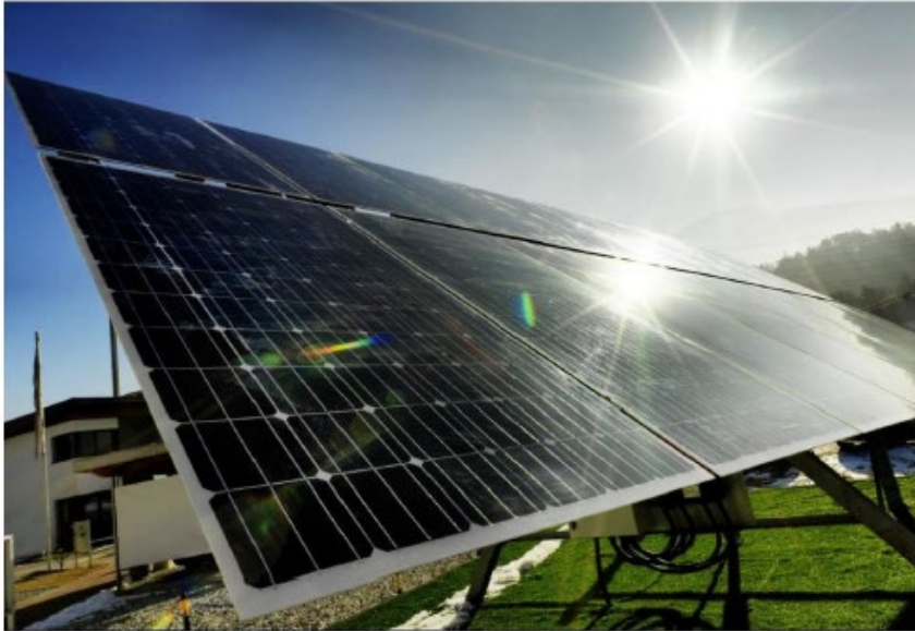
Solar panel showing solar glare
