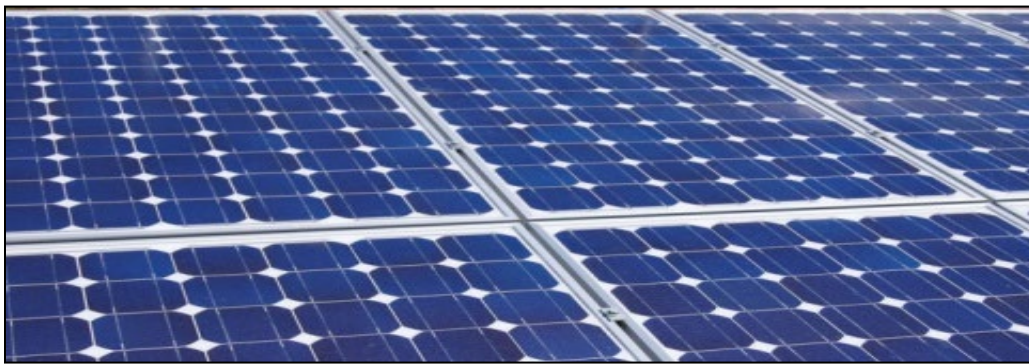
Figure 11. Module Spacing Gaps
